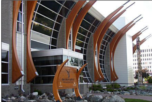
Building in Prince George, BC.
