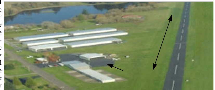
7S9 looking north. Arrows indicate the grass runway and Main Hangar BBQ, aircraft parking on the north side of this hangar.
